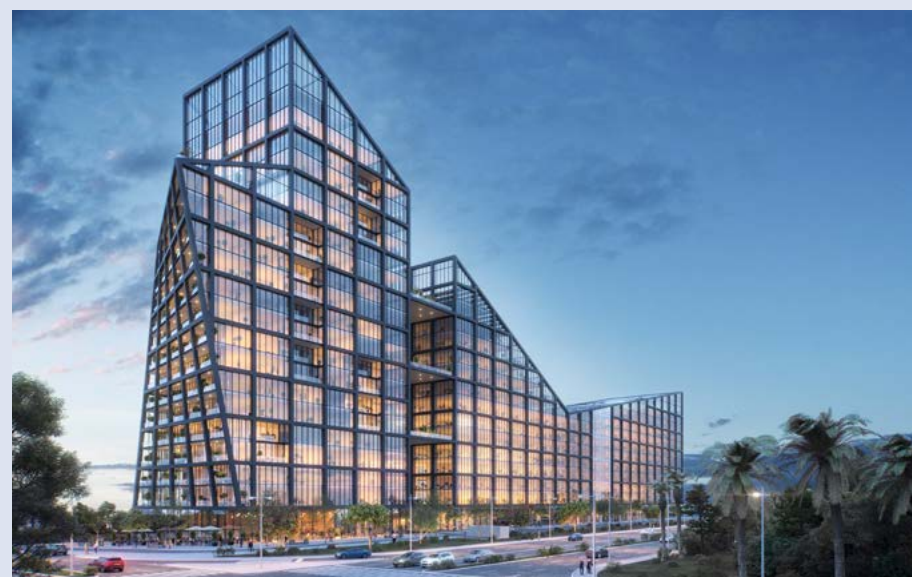
Matam East Towers #3
