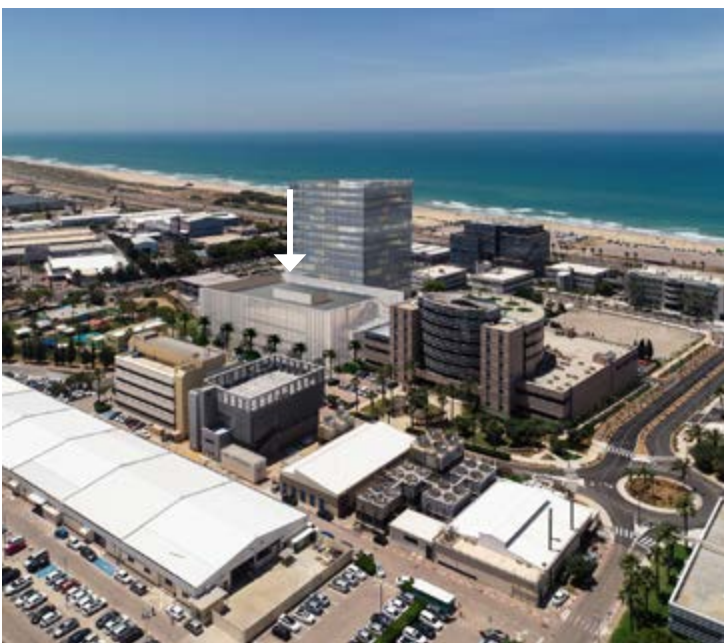
Server Farm 14,000 sqm (at MW10 supply) 100% marketed
