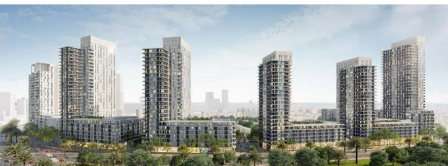
Tel Aviv - Dafna Project - Urban Renewal 360 units (company's share)
