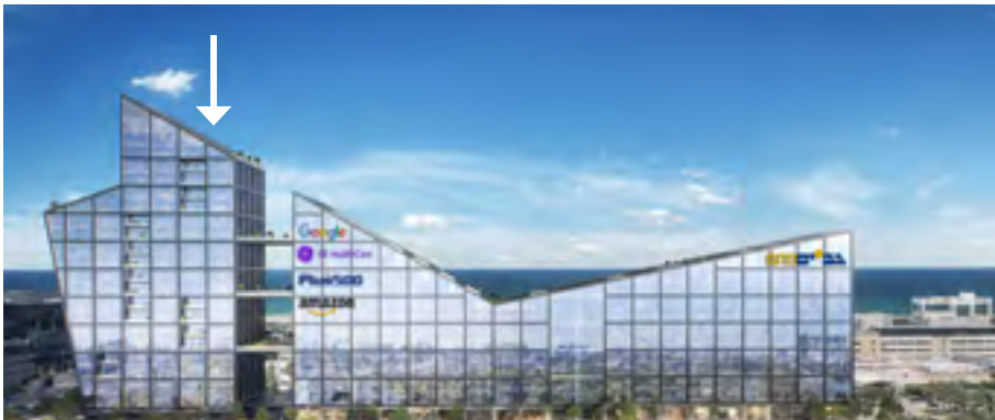
Matam East Towers #3 43,000 m2
